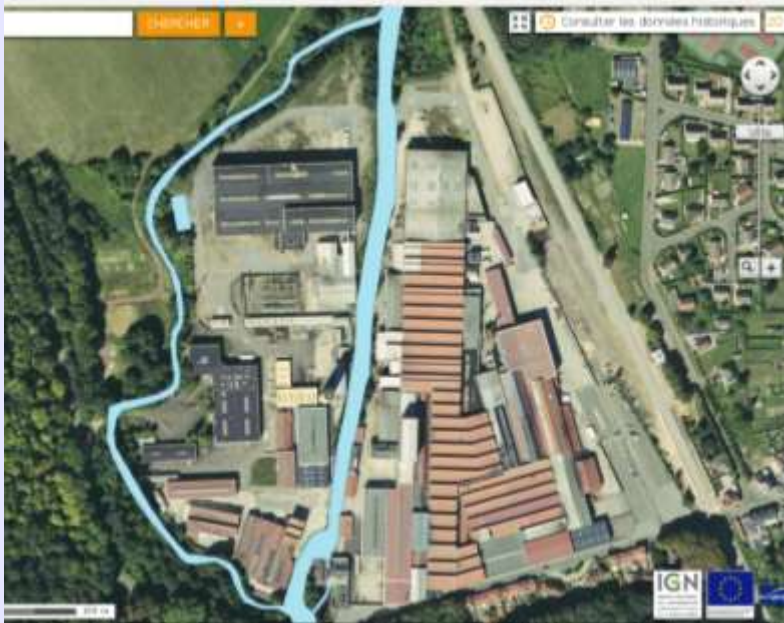
2,5MWp Solar Plant 2,8MWp Solar Plant
