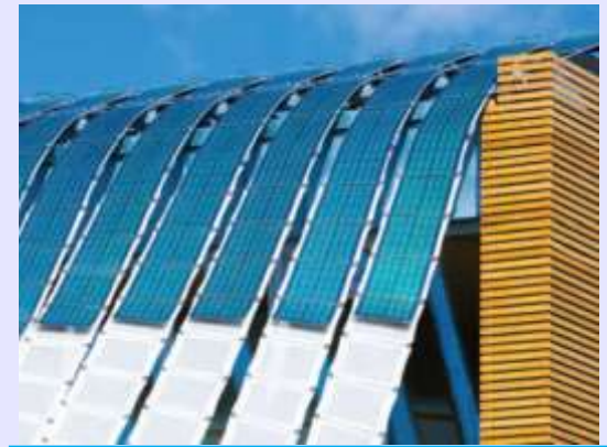
Solar Building integration
