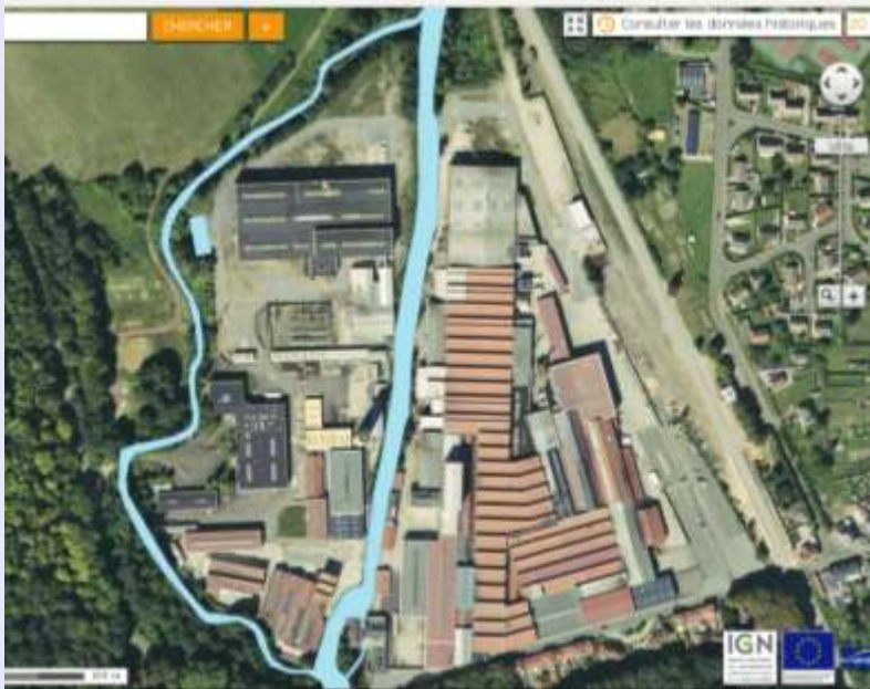
2,5MWp Solar Plant 2,8MWp Solar Plant
