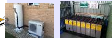
combination with CHP, heat pump, battery pack, rain-water install...
