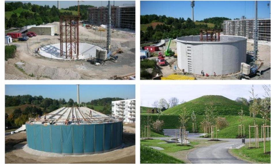
Construction of the seasonal heat storage in Munich, 5700 m 3 , 2007
