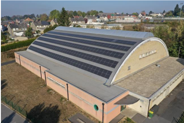
Gymnase Léo Lagrange
