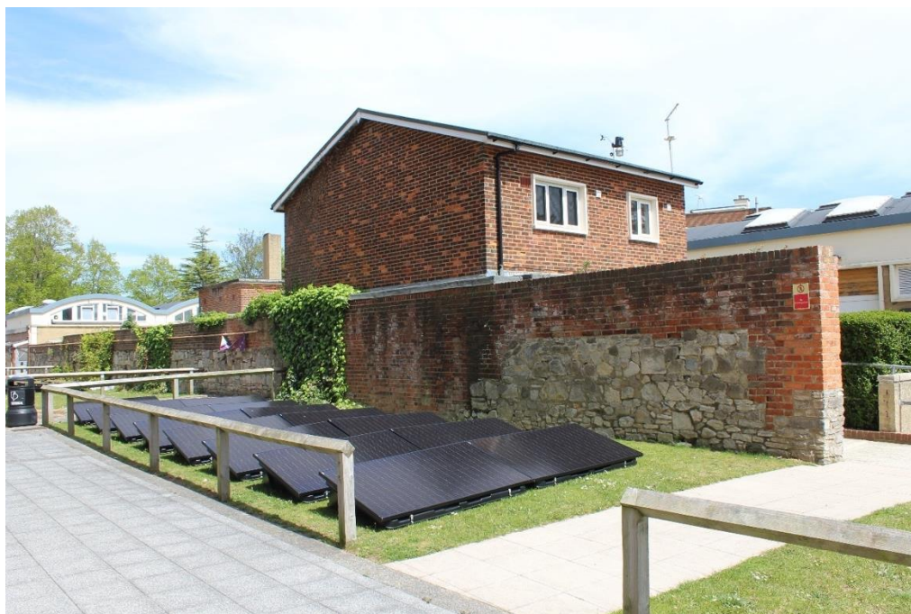
Figure 3: This image shows the installed 5kW photovoltaic solar array on the adjacent lawn by the Port-Eco House, which is shown to the right of the panels.
