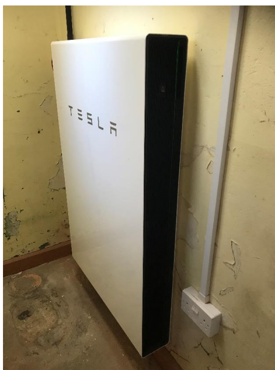
Figure 4: The image shows the Tesla Powerwall 2 battery that was installed in a storage room at the back of the Port-Eco-House.
