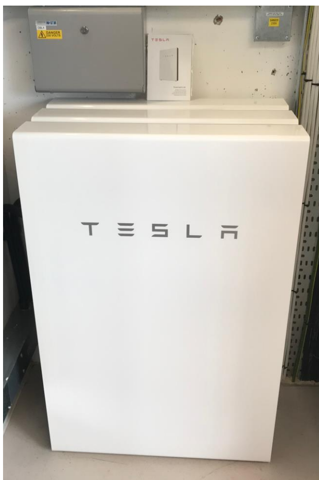
Figure 6: The image shows a bank of three Tesla Powerwall 2 batteries installed at the Future Technology Centre with a total energy storage capacity of 40.5 kWh.
