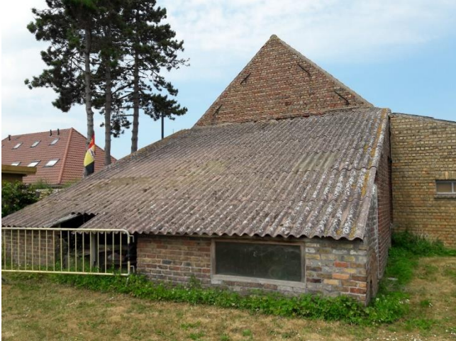
Figure 1: Roof with asbestos next to Groenhagemolen, before renovation
