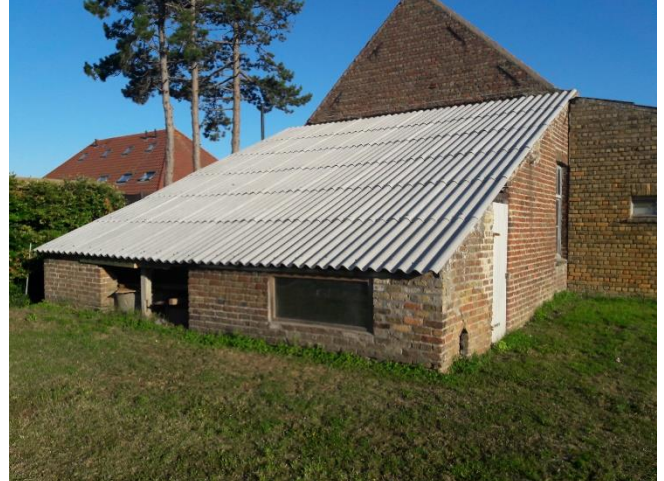
Figure 2: Renovated roof for PV installation
