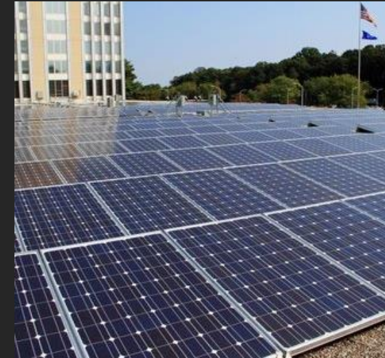
NIST rooftop, Maryland, USA [2]
