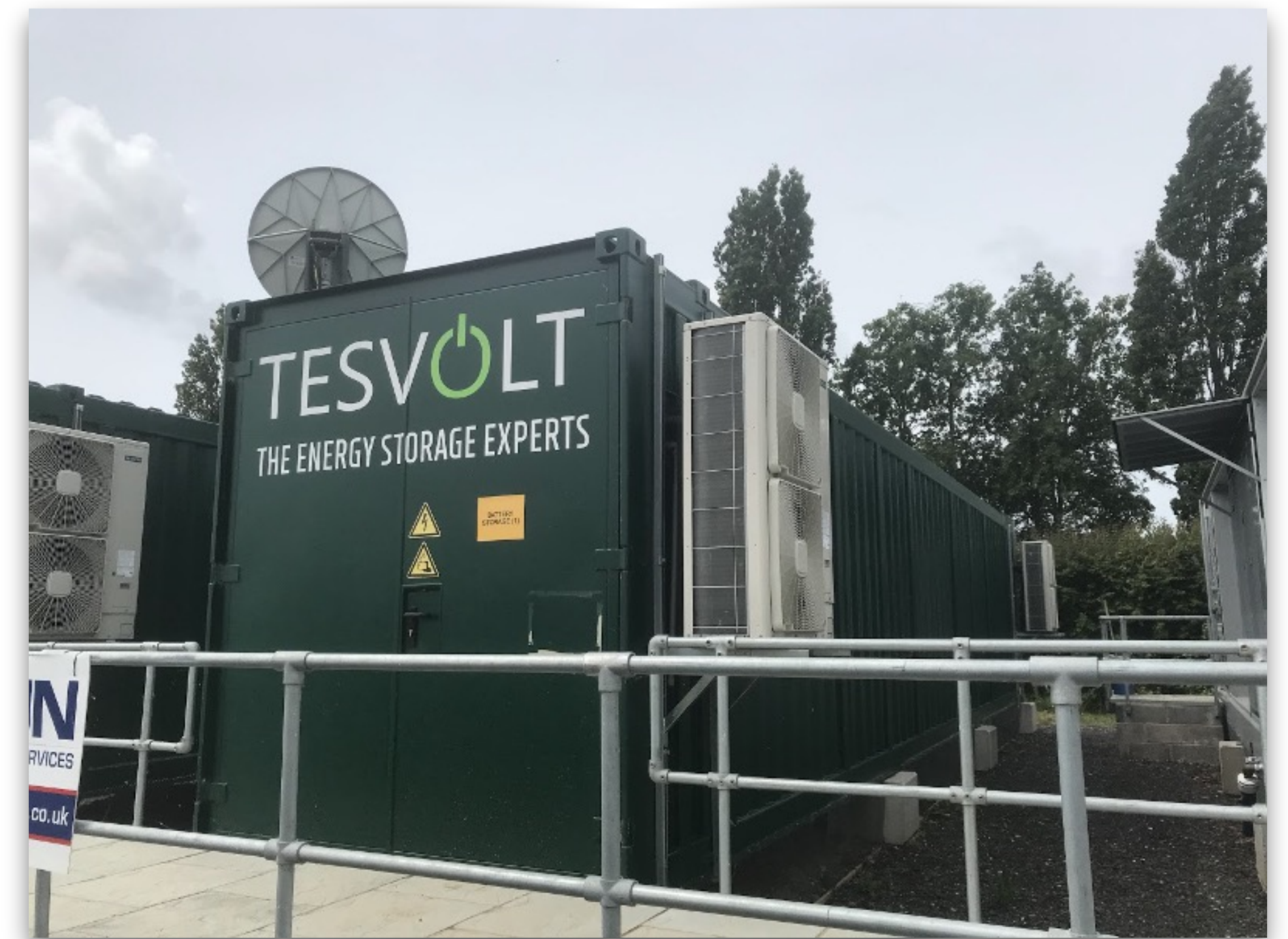
Grid-scale 2 MWh Lithium-Ion battery storage container at Westhampnett solar farm in West Sussex, England.
