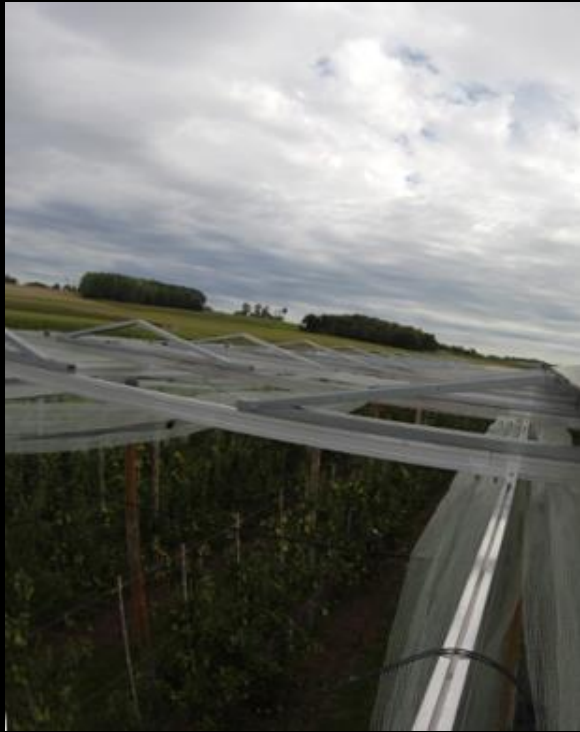
Aluminium frame on poles with L-profiles
