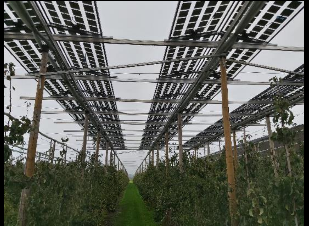
Rigid lateral wind bracing
