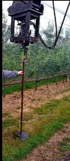
Soil anchor positioning
